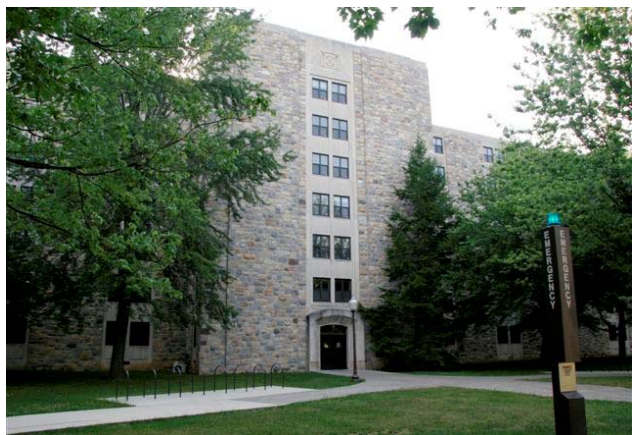
Figure 3. Exterior of West Ambler Johnston
